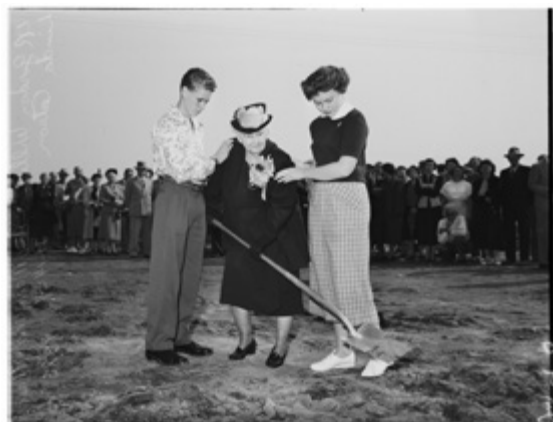
Ground breaking for Whaley Middle School, 1951
