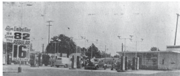
Gas station on Compton Boulevard, two blocks west of Atlantic Avenue, 1950
