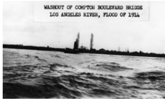
Los Angeles River in flood. Compton Boulevard Bridge washout, 1914
