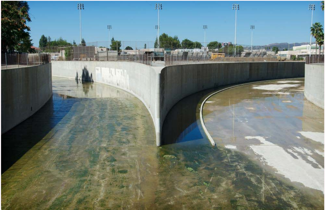
Fig 4. LA River Headwaters
