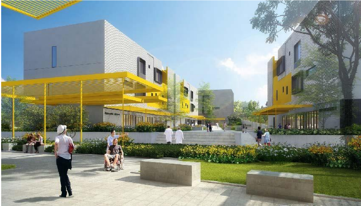
Fig. 2: Conceptual Rendering of Exterior Spaces for LAC-USC Restorative Care Village by NAC Architects.
